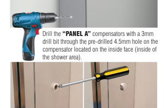
Using the screws supplied in **Pack "A"** securely fix both panels to the wall compensators and conceal using the supplied chrome cover caps .
