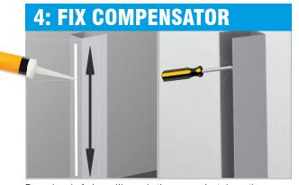
Run a bead of clear silicone bathroom sealant down the narrow face, for the full length of the outer compensator and then screw to the wall using suitable screws (**NOT SUPPLIED**). Wipe **ANY** excess silicone from compensator/wall joint.
