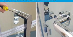
Offer an external handle to the outside of **PANEL "C"**. Attach the remaing internal handle to the reverse of **PANEL "C"**
