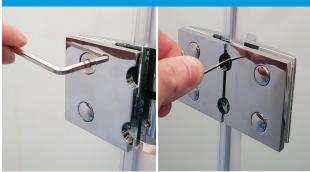
With **"PANEL D"** in the closed position, use a 5mm allen key to tighten the 4 x allen screws on each hinge, see above left. Attach the 4 x chrome cover caps to cover the screw heads.
