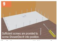
Use the longer screws provided to secure the ShowerDec® to the floor joists. Ensure ShowerDec® is secured along all 4 edges to eliminate any movement.
