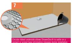
Carefully place ShowerDec® into position. Checking levels in both directions, gently tap ShowerDec® down until level on all 4 sides. It may be necessary to add more self levelling screed, do this by slighlty lifting ShowerDec® & pouring in the screed. Gently tap again until level on all 4 sides.
