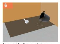
Apply a self levelling screed mix to cover all of the proposed area. This will ensure ShowerDec® is fully supported. **Caution!** Ensure the void around the trap
